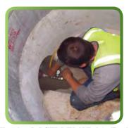
Typical ASTM F1417 Air Test
